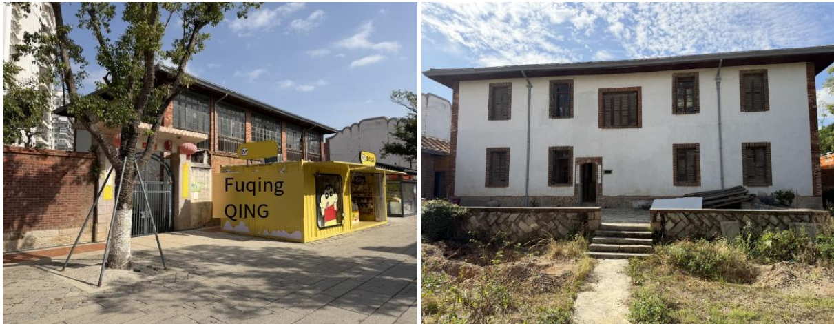
Figure 6: Facade of the South Building. Left: front; right: back. (Source: Authors).
