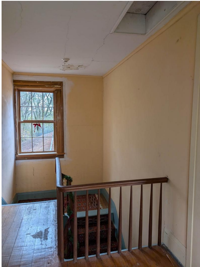
Figure 5: Staircase with the opening designed to improve ventilation. (Source: Author, November 2024).
