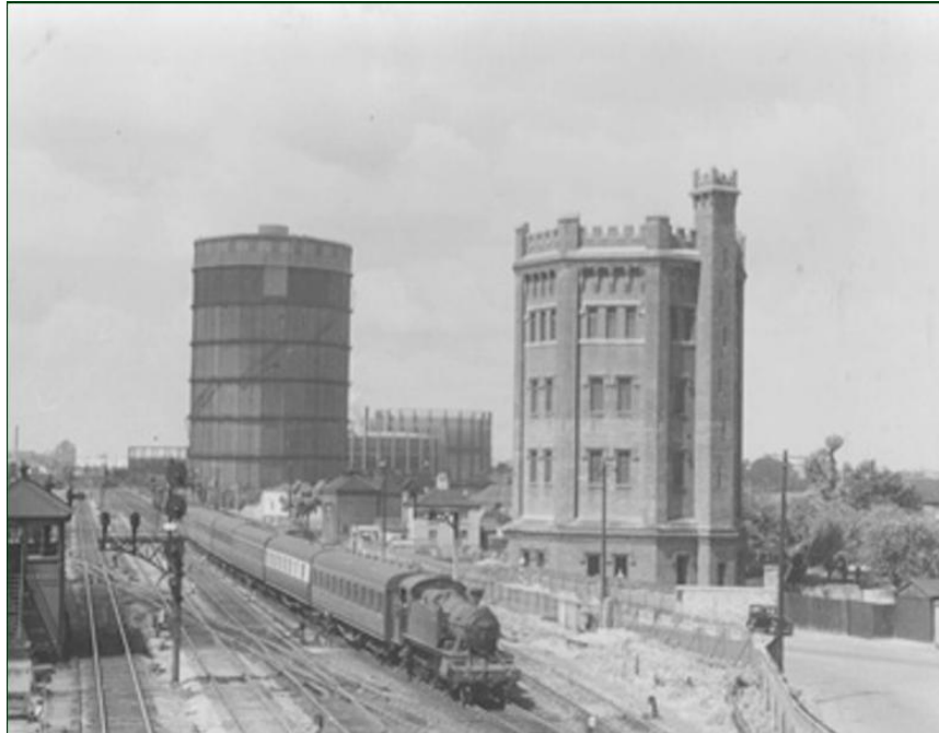
Fig. 4: Southall Water Tower (Source: Ealing Council, Southall Historical Walk Guide).
