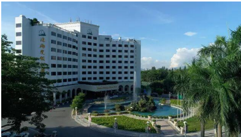
Figure 9: Main Building of Zhuhai Holiday Resort Hotel. (Source: Zhuhai Holiday Resort Hotel).
