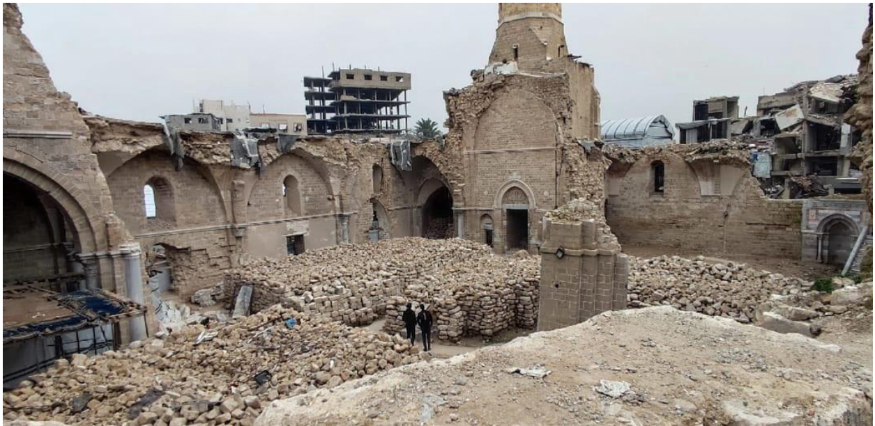
Figure 8: Beginning of restoration work of Great Omari Mosque in Gaza City including collection and sorting of its stones. (Source: Riwaq Photo Archive, 2025).
