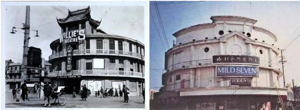
Figure 9: Comparison of the Victory Cinema tower before and after demolition. (Source: Shanghai Hongkou, "Shengli dianyingyuan bi 'ye' huigui, bainian jianzhu xiaomie 'shiwang huoji' | Genzhe biaoqingbao daka Hongkou ③" [Victory Cinema Returns with a 'V' Gesture, Century-old Building Eliminates 'Urgent Danger' | Check in at Hongkou with Emojis ③], January 31, 2025, accessed April 9, 2026 https://baijiahao.baidu.com/s?id=1822716830236670379&wfr=spider&for=pc ).
