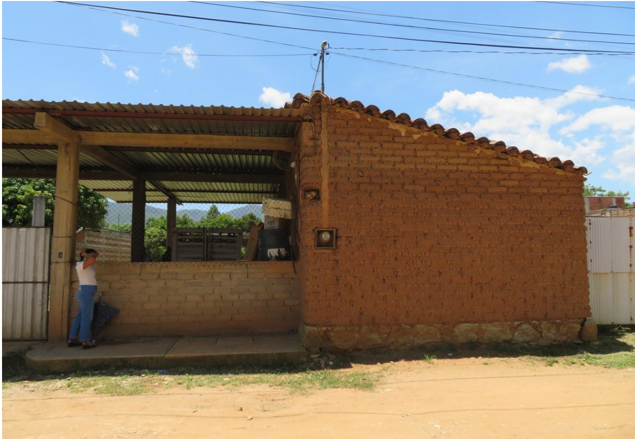
Figure 3: A typical, 50-year old adobe house in Santo Domingo Tomaltepec, which features a stone base and clay-tile roof, has been carefully maintained; the adjacent structure in concrete and metal was added in recent years. (Source: Catherine Sckerl, 2025).
