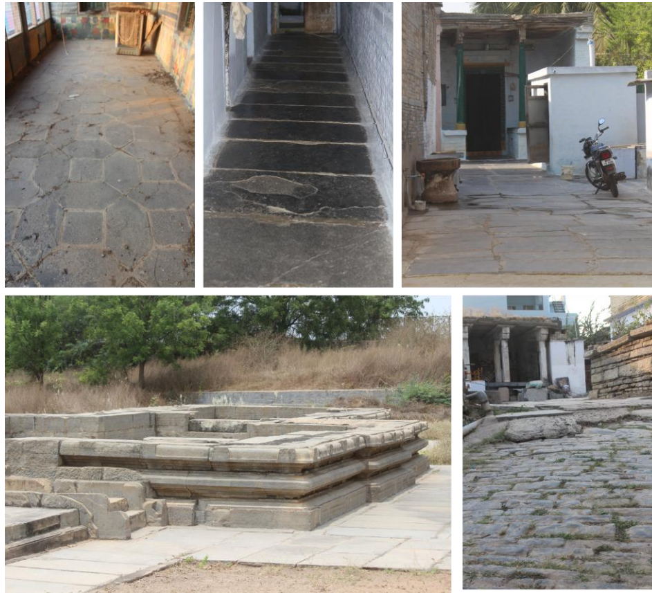
Figure 6: Indigenous techniques of flooring, pavement, and plinth construction. (Source: Authors).
