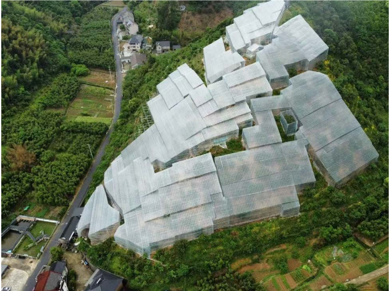
Figure 4: Bayberry greenhouses, Lin'an District, Hangzhou, China. Photograph by Kejia Mei, 2023. Comparable slope-adaptive techniques are found across Zhejiang, including in the more mountainous terrain of Wenzhou.
