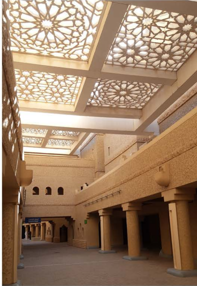
Figure 5: Residential Building in Diplomatic Quarter, Riyadh; the urban corridors are protected by a reinterpretation of traditional mashrabiya elements in concrete (Source: author).
