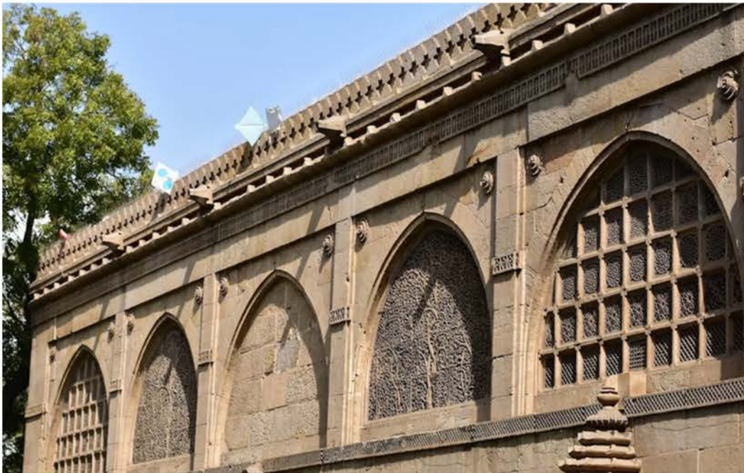
Figure 1: Sidi Saiyyed Mosque, façade featuring mashrabiya (Source: Mazzetto and Noca, 2025).
