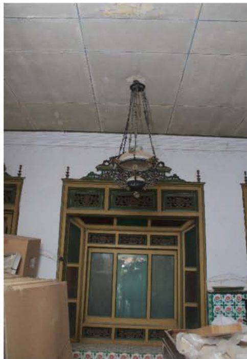
Figure 8: Ruang dalem is used as a wood storage (Source: Nanick,W. (2024)).
