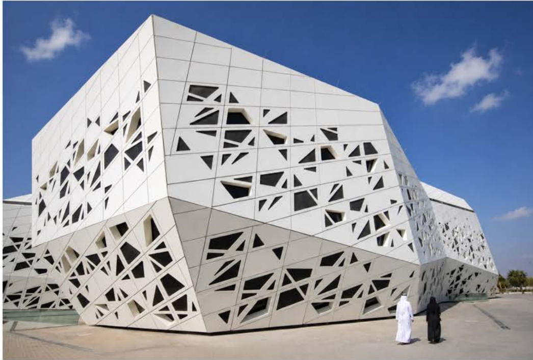
Figure 2: King Abdullah Petroleum Studies and Research Center, elevation showing the shading devices and reinterpreting the traditional mashrabiya in a contemporary, high-tech structure (Source: author).
