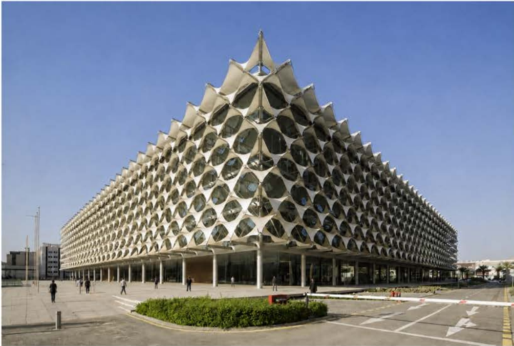
Figure 3: King Fahad National Library, Riyadh: elevations showing the textile shading devices fusing traditional architecture with a reinterpretation of contemporary design (Source: author).
