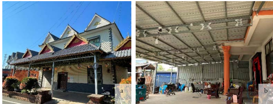
Figure 3: Column-supported canopy of brick-concrete houses (a) Two-tiered pitched roof form (b) Flat-roof form (Source: Authors).
