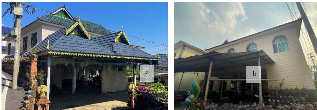
Figure 4: Column-supported canopy of concrete-frame houses (a) Two-tiered pitched roof form (b) Flat-roof form (Source: Authors).
