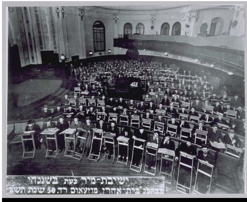
Figure 3: Interior View of Beth Aharon Synagogue
