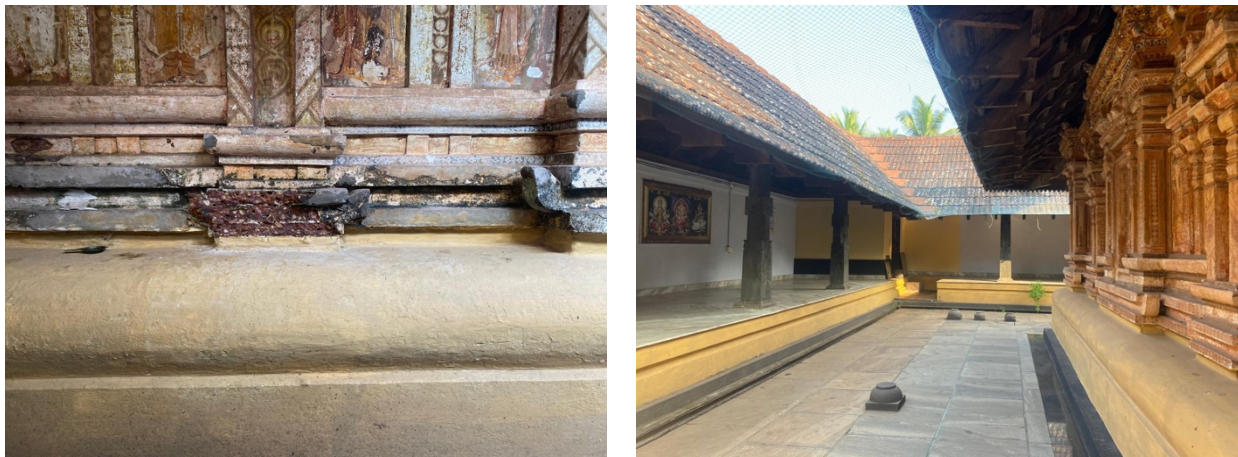
Fig. 3. Laterite stone walls in Chendamangalam Temple, Vadakara. Image source: authors
