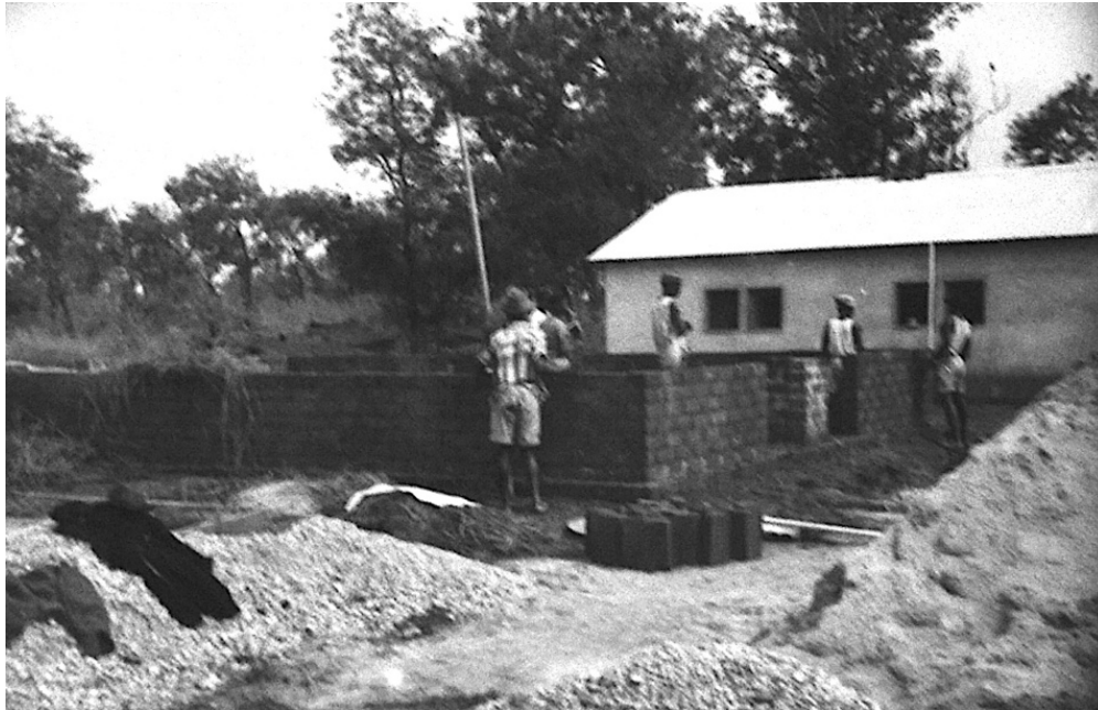
Fig. 6: “Experiments with earth blocks in the village of Chilupuca”, Lunda, 1954 (Source: DCV-UC/AD).
