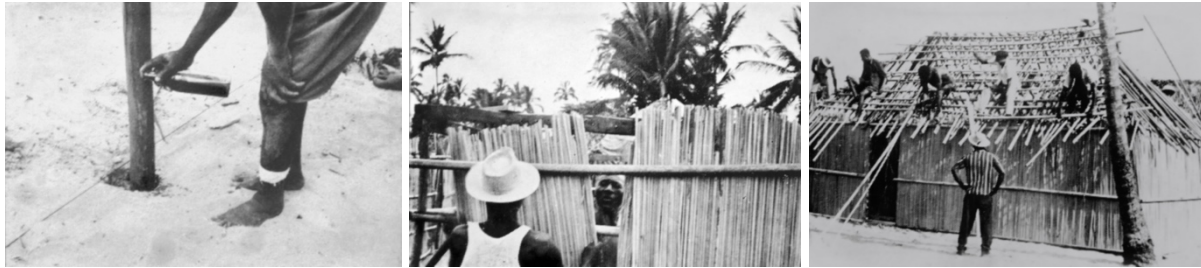
Fig. 4: Stages in the construction of Casa Axiluanda : ceremony of pouring wine into the jitungu ; building walls with luandos ; framing the roof with coconut tree slats. (Source: Fernão Lopes Simões de Carvalho, Contribution à l'étude du renouvellement des groupes d'habitations des pêcheurs de l'Île de Luanda-Angola , c. 1965, p. 46 and 53. Courtesy Inês Lima Rodrigues).
