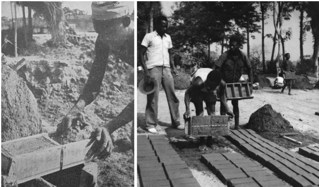
Fig. 8: “This brickmaker has already filled and scraped one half of his mold”, Belgian Congo (Source: A Chacun sa Maison , 1953, 28); “Dundo brickworks [Lunda]. Brick molding using quadruple forms”, 1955 (Source: DCV-UC/AD).
