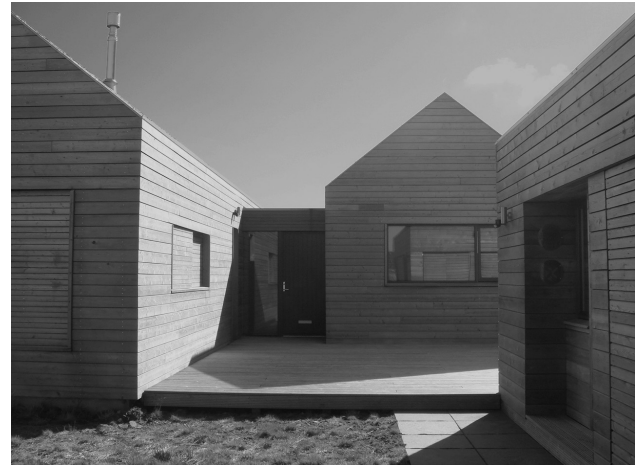
FIGURE 11. Dualchas Architects have increasingly used as-found, or “brut,” materials in their work, as demonstrated by the larch-plank rainscreen on the house at Boreraig. Photo © the author.
