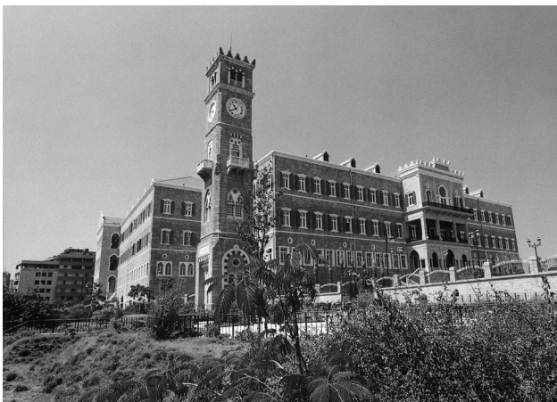
FIGURE 10. The Grand Serail. TOP TO BOTTOM: the building as it appeared in its original form, during the civil war, and as a postwar reincarnation. Source: Ayman Trawi.
