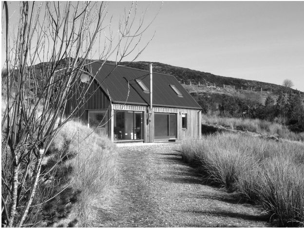
FIGURE 7. Larch Cottage, Drumfearn, Isle of Skye, designed by Mary Arnold Foster of Dualchas Architects, adopts a long, low form that echoes the proportions of the blackhouse, and that is sited carefully in a natural hollow that protects it from the prevailing winds. Photo © the author.
