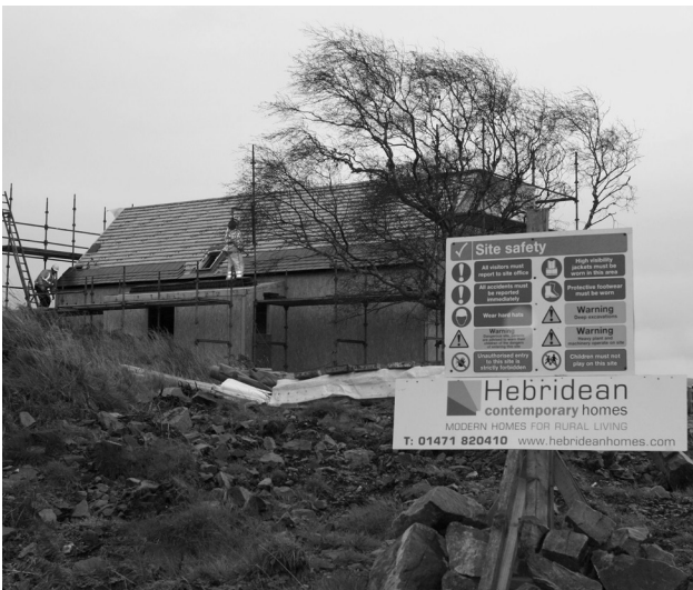
FIGURE 17. An LH102P design taking shape at Kilnaish near Tarbert in Argyll. This is one of the standard house types that forms part of Dualchas Architects' HEBHOMES project. The project aims to provide low-cost housing that continues the longhouse typology. Photo © Dualchas Architects.
