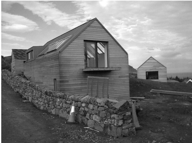
FIGURE 10. The house at Flodigarrry split the accommodation into three parts — a dwelling, an outbuilding, and a self-contained flat — and located the accommodation in three different-sized longhouse forms. These were sited on a hillside in positions that both minimized the necessity for earth-moving and optimized the aspect from the main buildings. Photo © the author.
