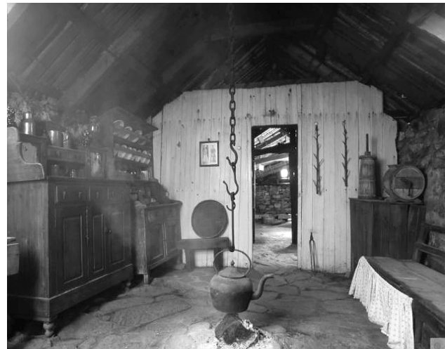
FIGURE 14. Reconstruction of a blackhouse interior at No. 42 Arnol, Lewis (c.1885) (owned by Historic Scotland), showing the single living space with its central peat fire. Photo © Crown Copyright, reproduced courtesy of Historic Scotland, www.historicscotlandimages.gov.uk .
