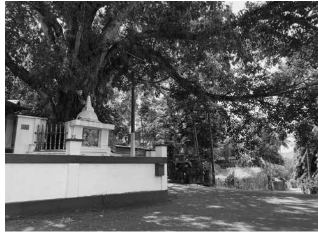
FIGURE 13. Overall view of Watapuluwa Housing Scheme, Kandy. Photo by author, 2023.
