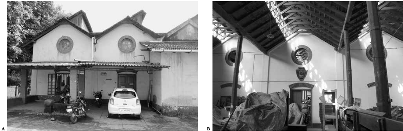
FIGURE 8 (A AND B). Contemporary exterior and interior views of the printing press building in Mangalore, used as a printing press in 2018. Photos by author.
