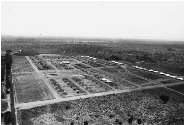
FIGURE 3. The construction of the Ajuda neighborhood, aerial view (1965–1966). Photo courtesy of Prof. Sandra Mula.
