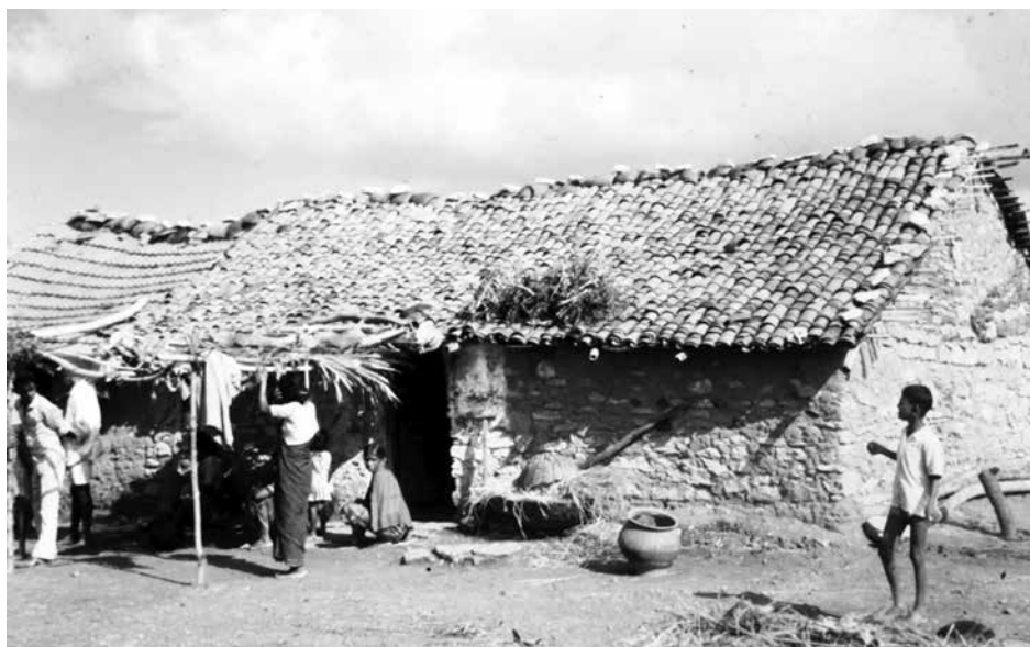
FIGURE 1. A potter's house in rural Karnataka, which is roofed partly with country tiles and partly with Mangalore tiles. Source: Dr. Kaup Jagadish, 1980.
