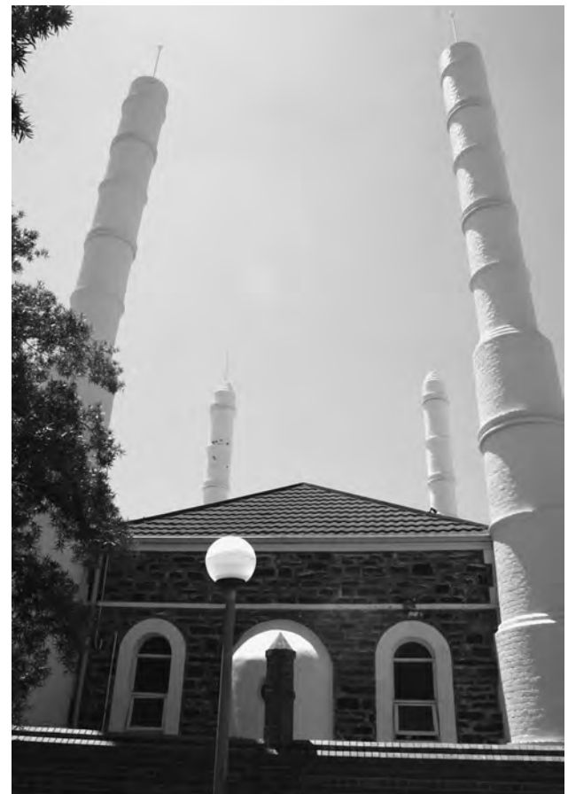
FIGURE 10. The Adelaide mosque in its current state, showing its bluestone masonry, mihrab, arched windows, and four minarets. Photo by Mizanur Rashid, 2012.
