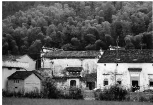
FIGURE 1. The lime-plastered Yin Yu Tang house (center) in its original setting in Huang Cun. Source: N. Berliner, Yin Yu Tang: The Architecture and Daily Life of a Chinese House (North Clarendon, VT: Tuttle Publishing, 2003), p.32.
