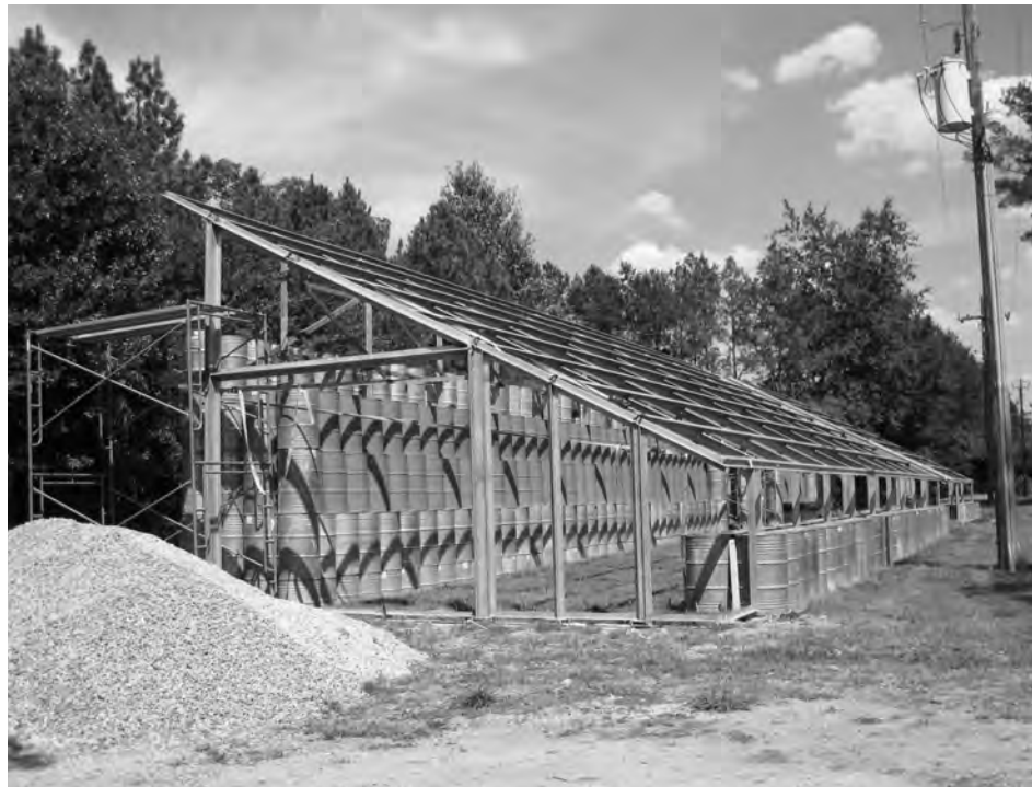
FIGURE 13. Rural Studio greenhouse (under construction), 2011–2013. Photo by author, fall 2014.
