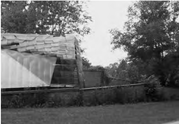
FIGURE 7. Mason's Bend Community Center/"Glass Chapel," Samuel Mockbee (studio director) and students of the Rural Studio, 2000. Mason's Bend, Hale County, Alabama. Built with recycled windshields and rammed earth. Photo by author, summer 2010.
