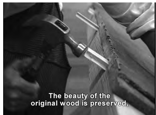
FIGURE 3. A close-up from the documentary film Yin Yu Tang: A Chinese Home showing how two boards are joined using a traditional dovetail tenon. Courtesy of the Peabody Essex Museum.
