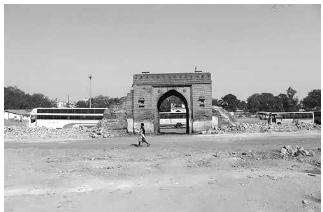
FIGURE 16A, B. The enclosure near Astodia Darwaza built during Mughal rule that was used as a leper asylum during colonial rule. Part of the enclosure was demolished recently in preparation for the expansion of the Geeta Mandir bus depot.
