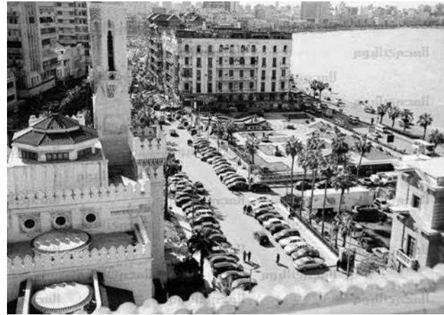
FIGURE 3. A view of the square before its redevelopment. Source: N. Abu Shal, “Alexandria: Commander Ibrahim turned into a Garage [al Āskandryāfī: al Qā’yd Ābrāhiym Taḥawal ila Ġaraġ],” al Masry al Youm, Cairo, January 24, 2016.
