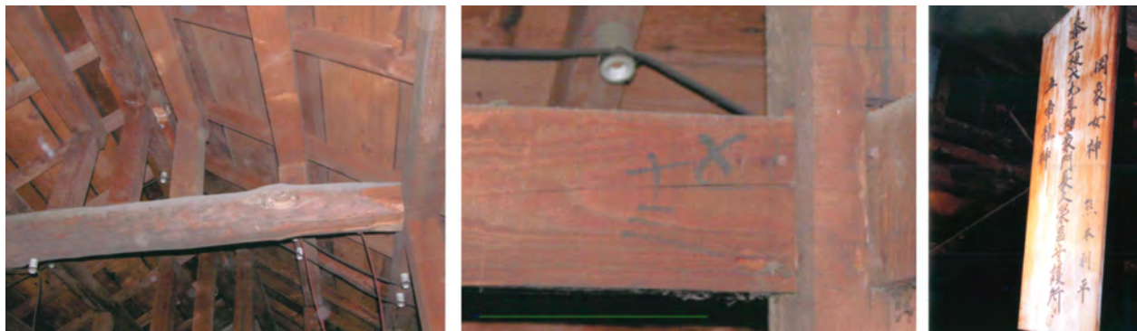
Figure 7. Traditional Japanese construction methods in the roof structure (left,) Bantsuke 36 Marking (center) and Munahuda found in attic.
