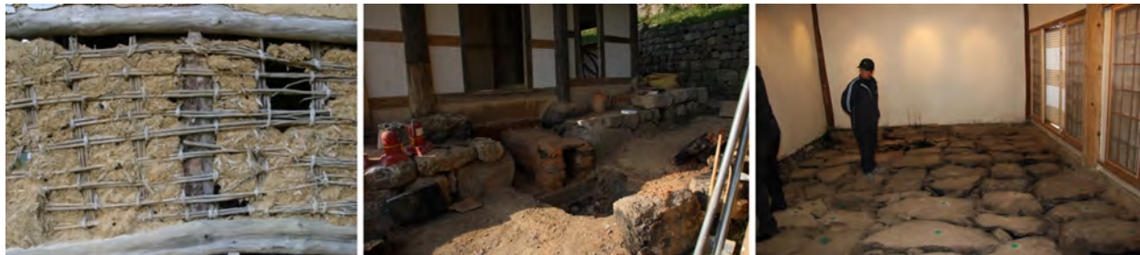
Figure 3. Inside of Ondol structure. Left is showing the inside of the soil wall. Middle is the fireplace, Agoong-i, is under construction. Right is Installation of Gudle stone. Smoke would go under these stones and heat the floor. Soil would cover later.
