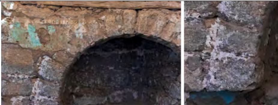
Figure 16: Mud bricks and mud in between the bricks
