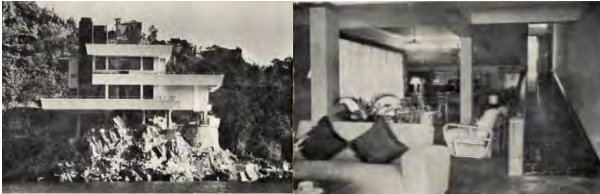
Figs. 14 (left) and 15 (right) The iconic Arrowhead (1953) (left) at Deep Water Bay, Hong Kong, with a ramp installed in place of conventional staircase, connecting the living room to the lobby and lobby to the master bedroom suite (right). It was described as the most unusual but outstanding feature of the building's interior. (Source: Hong Kong & Far East Builder, November & December 1953, 21-22)
