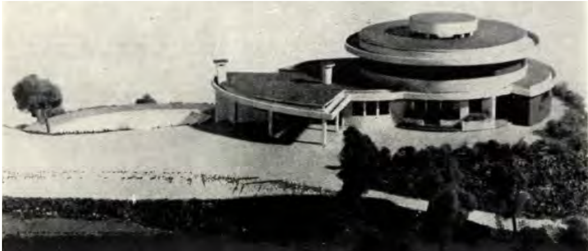
Fig. 19 An architectural model of Dr Carey-Hughes' Residences, with its main entrance pictured on the right. While a circular building requires the least walling, founding and roof in theory, it is particularly challenging to design one in reality given the propensity for awkward floor layout. (Source: Hong Kong & Far East Builder, March & April 1956, 13-14)
