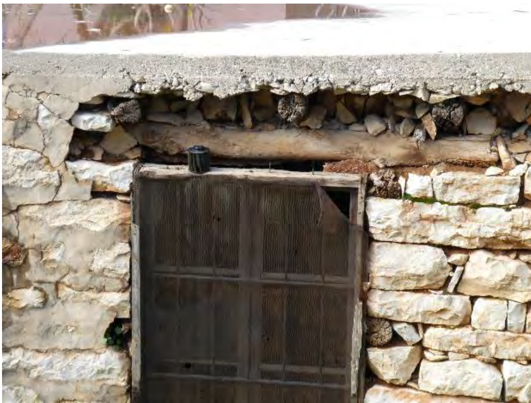
Fig. 5. Entrance photo showing the concrete intervention over the wooden ceiling (Source: Author, 2018)
