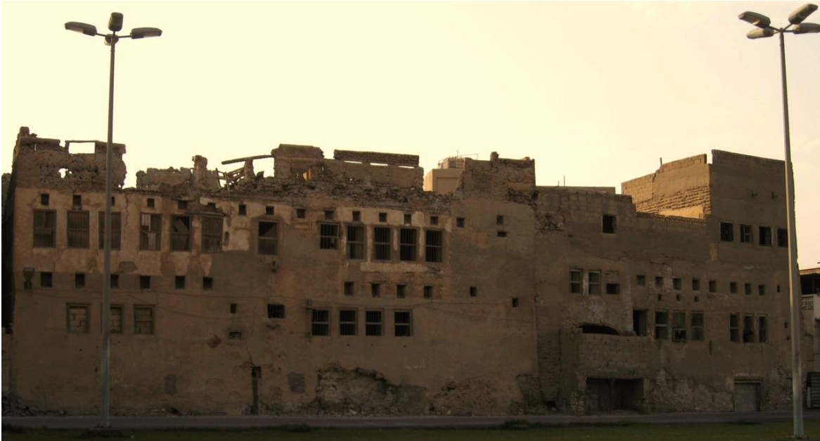
Fig. 8: Openings above eye level on the exterior façade to preserve privacy while allowing cross ventilation. (Source: Fieldwork by the author)
