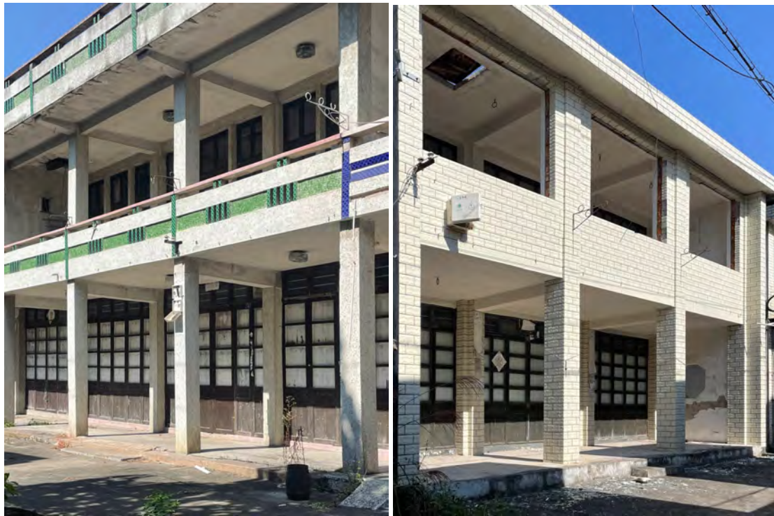
Fig. 6: Façades modifications using cement (on the left) and ceramic tiles (on the right). Both are cladding the exterior brick pier. Reinforced concrete structures replaced the wood beams and stone lintels. (Picture by Huang Tieru)
