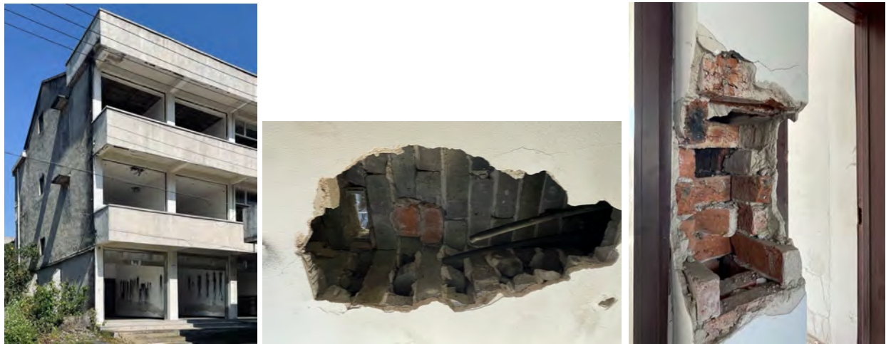
Fig. 7: Elevation of the house from two to three stories using the original grey kiln brick on the ground floor and fired red brick on the second and third floor (Picture by Huang Tieru)
