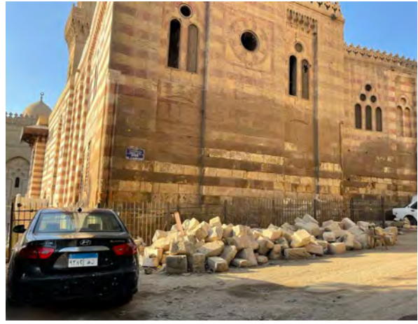
Fig. 7: Recent photo showing unrestored side façade with water damage and cracks. Finished front facade is the side on the left. (Photo by author)
