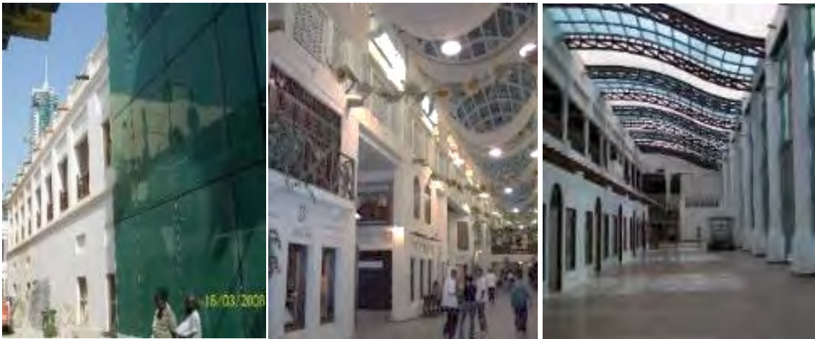
Fig. 20: Development of the new Souq in the traditional town of Manama-Bahrain; using extensive skylight of steel glazed ceiling. Increase the heat load and energy consumption with no care of sustainable environment building comfort (2006).
