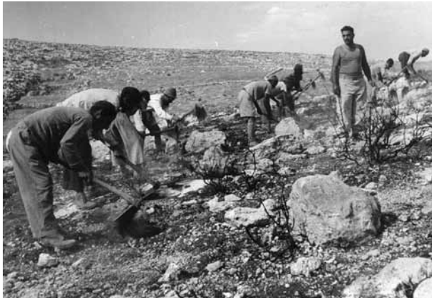
FIGURE 12. Ksalon: employment of dwellers in stone-clearing, 1950. Photograph by Werner Brown. Source: JNF archive, reprinted by permission.
