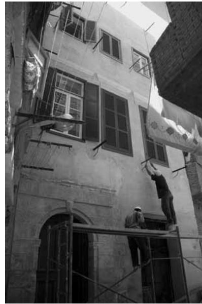
FIGURE 11. Renovated building facade in Atfet Hozayen, al-Darb al-Ahmar. The photo shows the clear modular style and the retained ground-floor stone-arch entrance. Courtesy of Aga Khan Trust for Culture, 2009.
