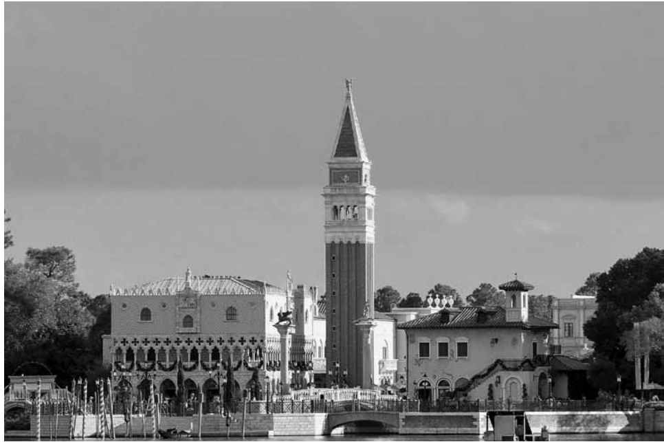
FIGURE 5. Italy Buildings in Epcot Theme Park, Orlando, Florida. Courtesy of Thomas Grim.
