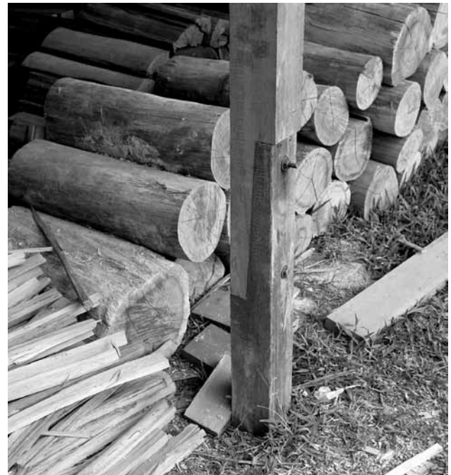
FIGURE 8. Nonlocal belian hardwood foundation post, cemented in and bolted to locally sourced hardwood upper structure. New house construction, Pa' Dalih, 2009. Photo by author.
