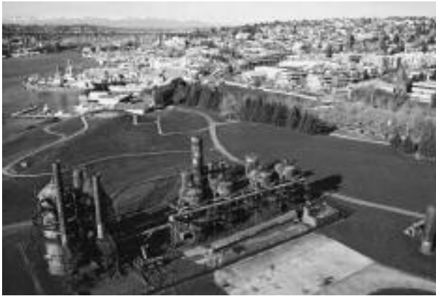
FIGURE 1. Gas Iron Works, Seattle, WA. Photo courtesy of Seattle Parks and Recreation.
