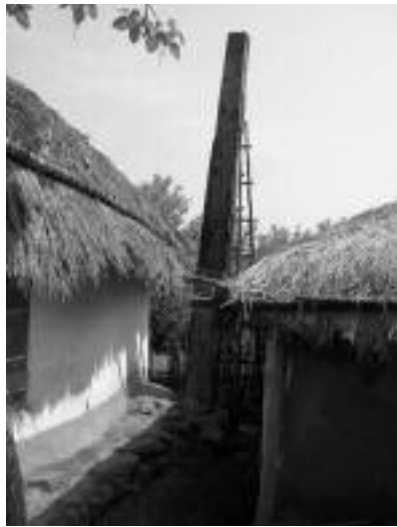
FIGURE 10. A Korean-Chinese chimney (Lutian Village) is built as a diminutive tower with a square vertical pipe, and is placed beyond the end-wall of the house.
