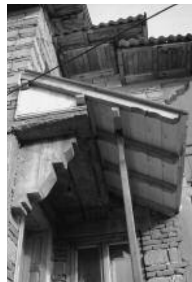
FIGURE 11 (ABOVE). The use of concrete to resemble the typical details of a timber structure, Corbsori village, Arges, 2007.
