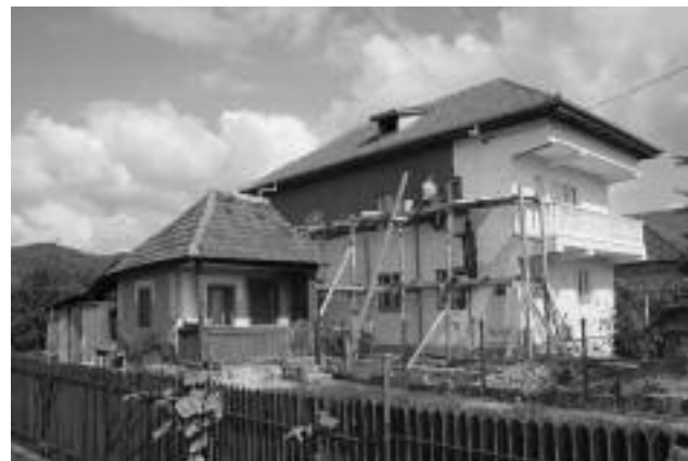
FIGURE 2. Erecting a new house in a village from Oltenia, 2007.
