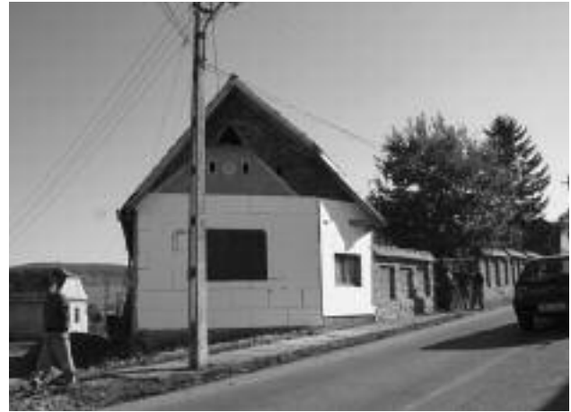
FIGURE 4. Polystyrene insulation used to blanket the walls of a beautifully decorated old house in a village from Sibiu, 2007.
