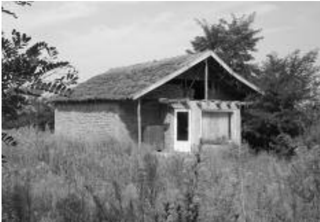
FIGURE 15. A new, unfinished house using adobe and thatch, but also thermal-insulating double-pane windows and doors. Topalu, Constanta, 2005
