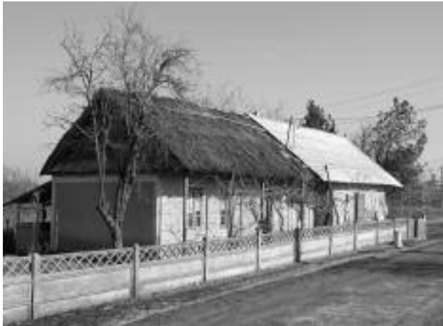
FIGURE 3. The use of reed thatch vs. corrugated metal sheets as a roofing material in the village of Murighiol, Tulcea, 2006.
