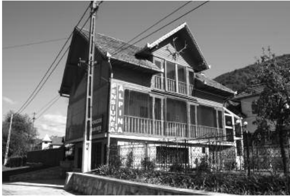
FIGURE 8. Agritourism: an example of a touristic pension where the typical open verandahs have been closed with glass (in front of the wooden structure), all around the house. Dragoslavele village, Dambovita, 2007.
