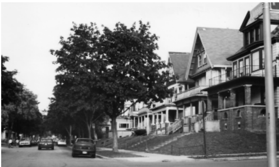
FIGURE 8. Large two-and-one-half-story duplexes built for German Immigrants between 1888 and 1910, rehabilitated by Hmong immigrants in the 1990s.
