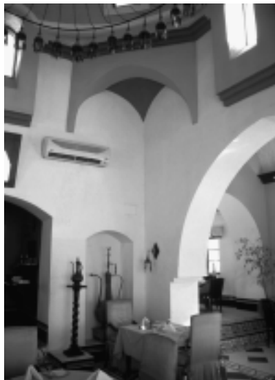
FIGURE 12. Air conditioning split units were eventually installed.
