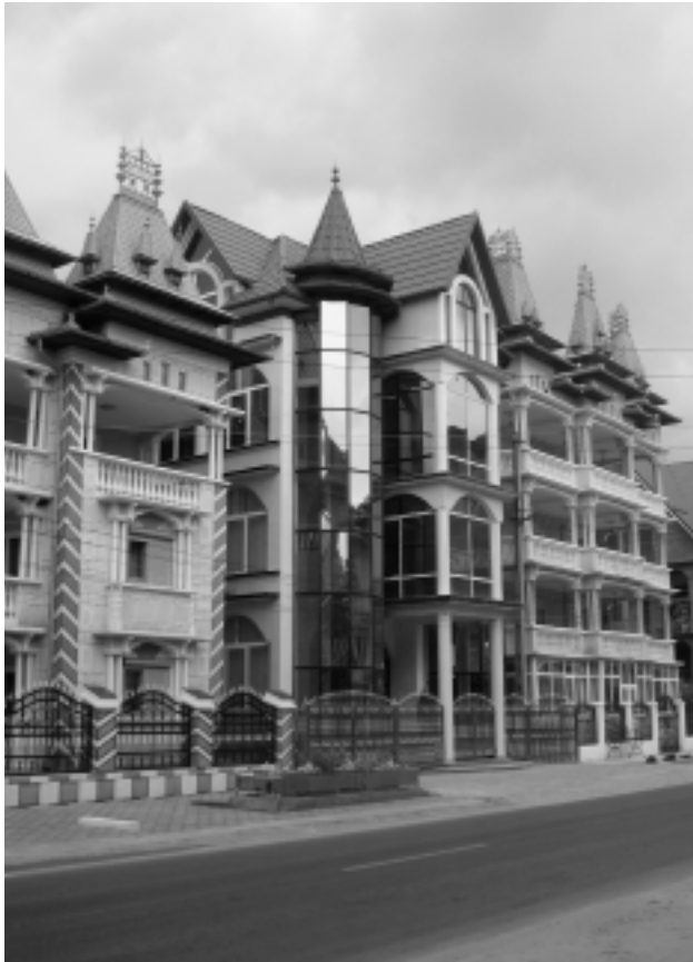
FIGURE 4. The glazed facade of a "palace" in Buzescu echoing the language of office towers in Bucharest.
