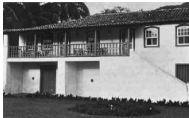
FIGURE 3. (BELOW) Example of Brazilian rural colonial manor house with elevated social rooms and front verandah.
