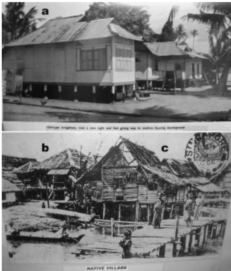
FIGURE 10. Historic examples of Malay-type houses in Singapore. (a) Gable-on-hip model (Bumbung Perak) from Geylang Serai area (caption: “Old-type bungalows, now a rare sight and fast giving way to modern housing development”). Source: Singapore Street Directory 1966. (b) Hipped-roof model (Bumbung Limas); and (c) gable-roofed model (Bumbung Panjang). Photo by author of a postcard, captioned “Native Village,” displayed in the Malay Village Gallery.
