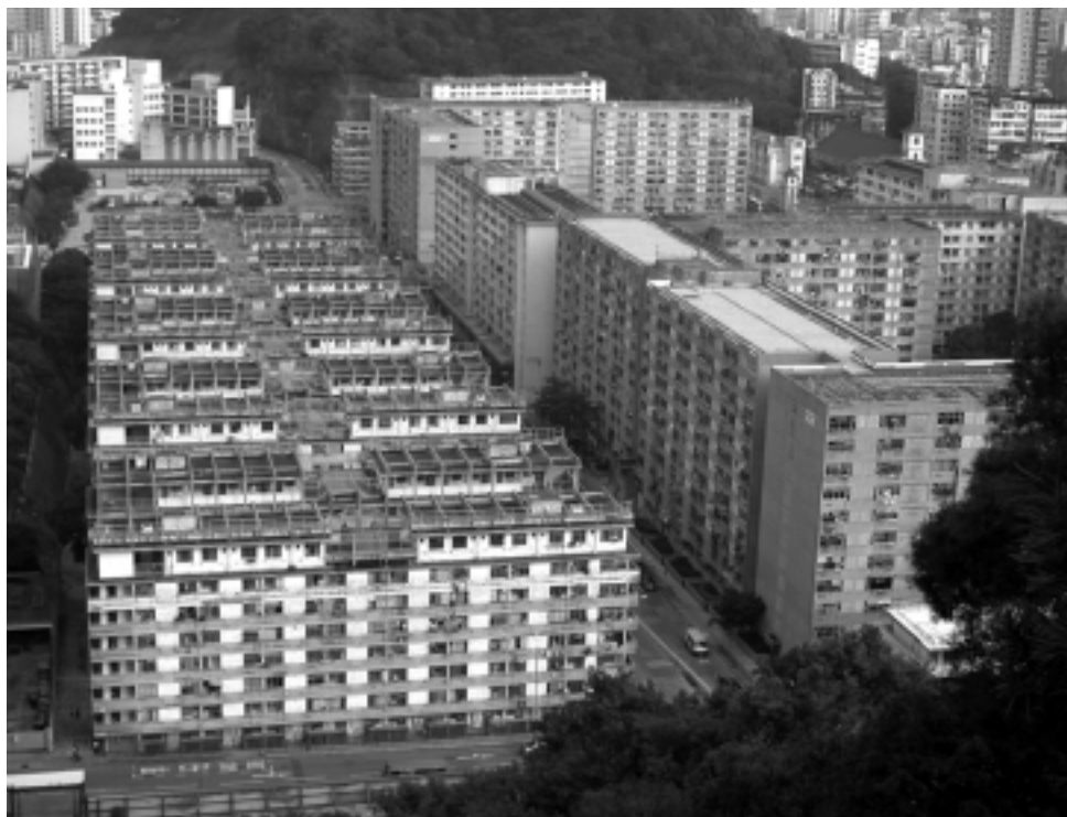
FIGURE 4. Birds-eye view of the Shekkipmei Estate showing different phases of its development.
