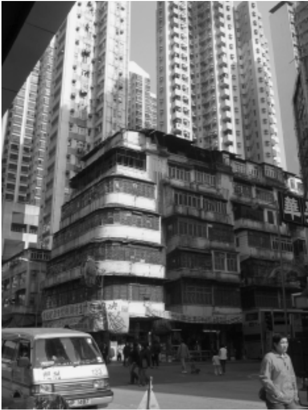
FIGURE 8. Urban landscape in Shumshuiipo showing an existing tenement building facing the fate of demolition. Many of these old tenements are located in districts that have been earmarked by the Urban Renewal Authority for redevelopment. Forced displacement resulting from this process had incited discontent among existing tenants and landlords. Note the banners on the building protesting the demolition. Photo by author.
