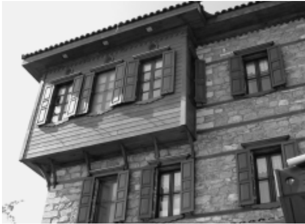
FIGURE 7. Restored house in Adatepe.
