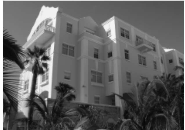
FIGURE 4. ACE Global Headquarters from the southeast. The architects were the Hillier Group of Princeton, NJ, with Harold Conyers and Associates of Bermuda.
