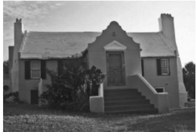
FIGURE 11. Oleander Circle, with a projecting entry porch, Flemish gable, and "welcoming arms" stairs. There are additional ells at the rear.
