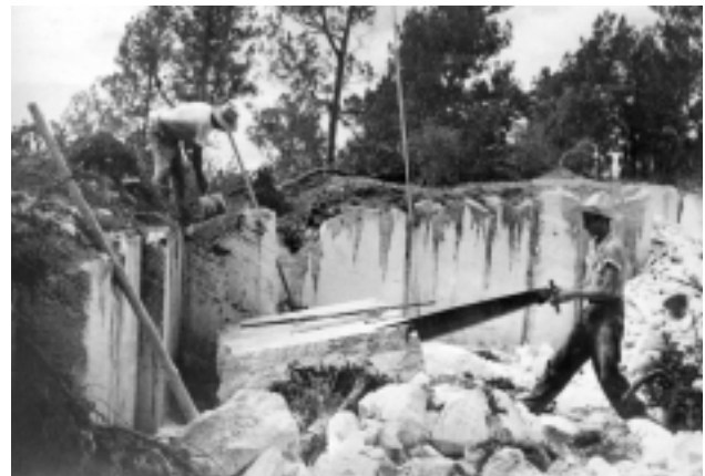
FIGURE 12. Bermuda's soft stone was once cut with handsaws. Archival photograph in the author's collection.
