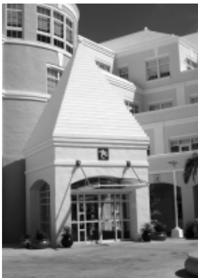
FIGURE 5. A) The ACE entry buttry. B) Bermuda’s eighteenth-century buttries, which still dot the landscape, were built for a variety of storage and food-related activities.
