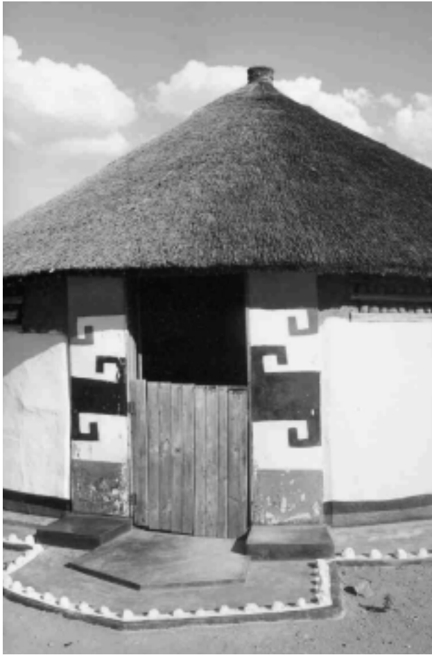
FIGURE 5. Example of isimodeni style (Type 3) building. Photo by author, 2000.
