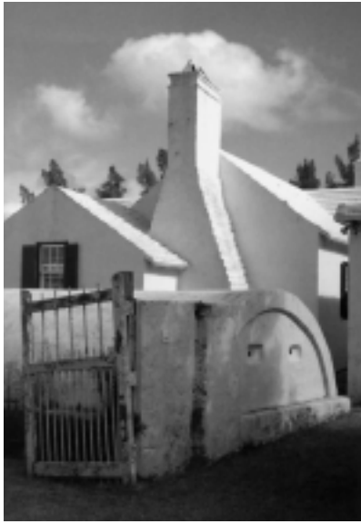
FIGURE 13. A domed water tank. Photo by Ian MacDonald-Smith.
