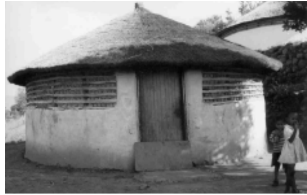
FIGURE 3. Type 1 Hlubi style building showing the open, packed eaves and painted, plastered walls. Photo by author, 2000.
