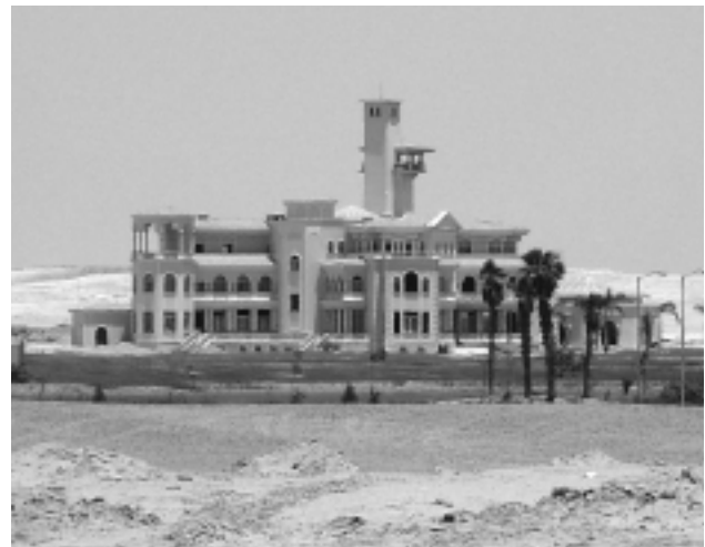
FIGURE 12. Initially, the principal shareholder wanted to build himself a replica of the White House, but eventually, he built a palace with a watchtower that overlooks the whole development.
