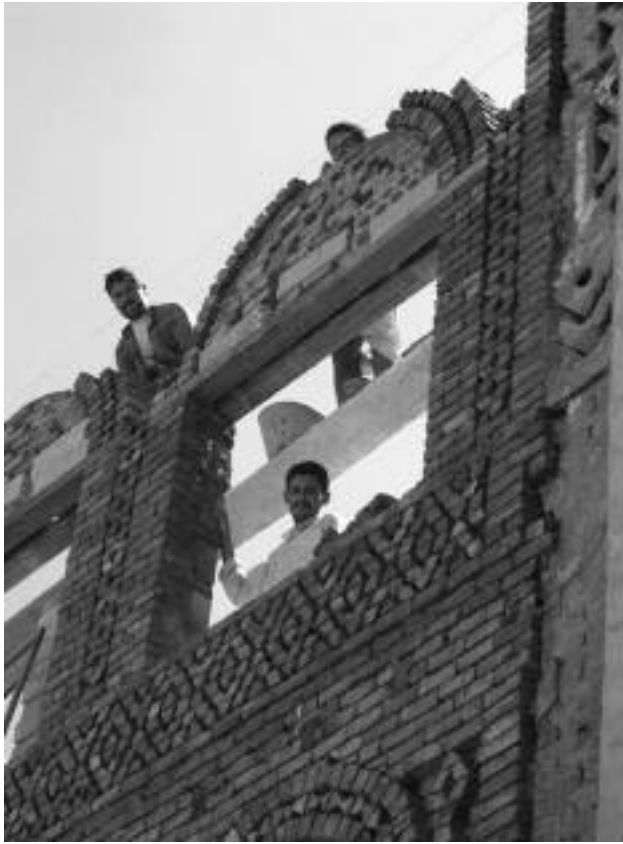
FIGURE 11. Brick arches and detailing applied as veneer on a concrete block wall.
