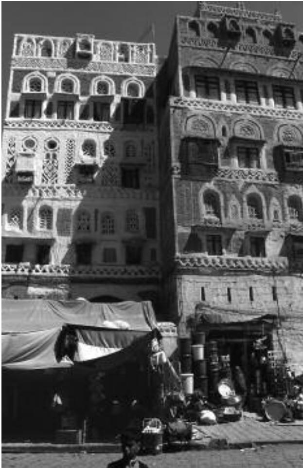
FIGURE 15. Shops installed in the ground floor of houses.
