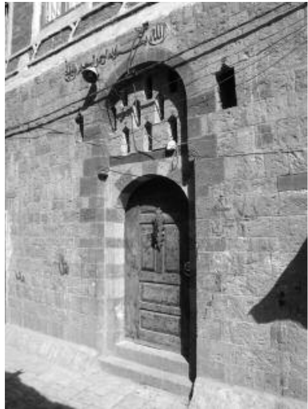
FIGURE 16 (RIGHT). A new door opening in a recent restoration, designed after the middle drawing in Figure 17 (the builder is the son of the usta whose work is shown in Figure 12).
