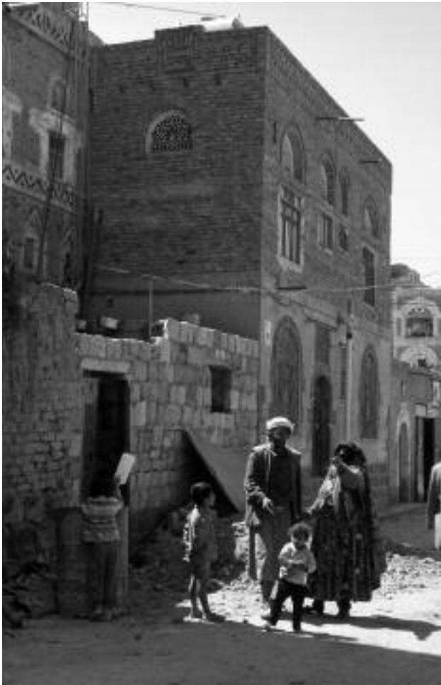
FIGURE 1. A woman in Sana'a furious at inspectors who are requiring her to dismantle a wall built in nonconforming materials.
