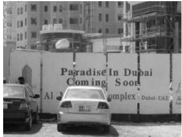
FIGURE 18. Construction site near Sheikh Zayed Road, Dubai.
