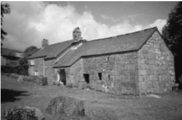
FIGURE 8. Sanders, a Dartmoor longhouse at Lettaford, near Chagford. The “livier,” or domestic end, is on higher ground than the “shippen.”
