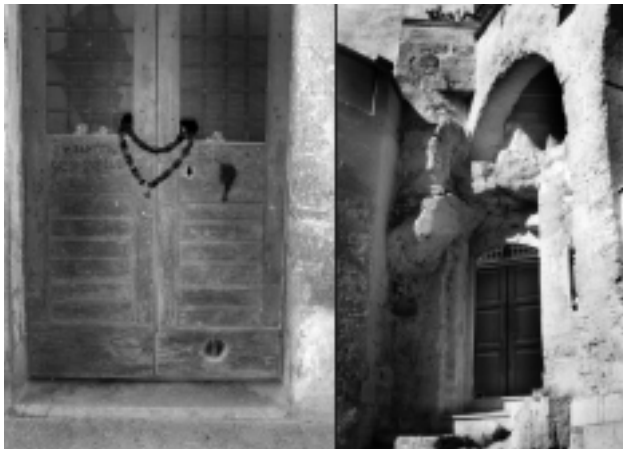
FIGURE 17. This pair of images compares an old, yet functional, brown door (left) with its cat door (blocked), and a new, industrially manufactured, green door (right) that complies with the Sassi preservation code. Left photograph by author, 2003; right photograph by Kathryn Toxey, 2000.
