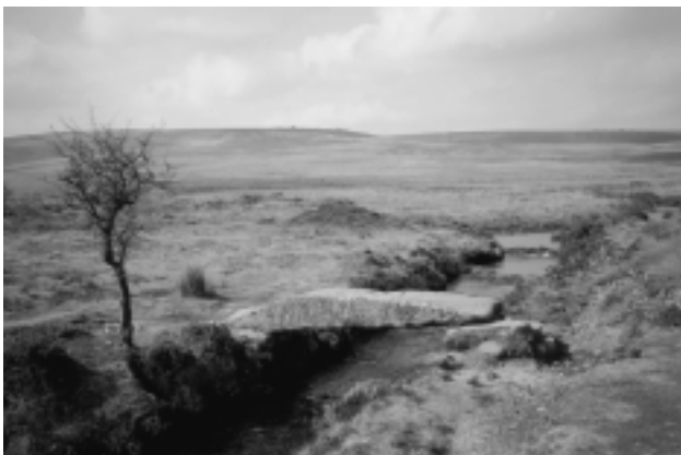
FIGURE 9. A Dartmoor granite monolithic clapper bridge crosses a “tinner’s leat,” or artificial stream.
