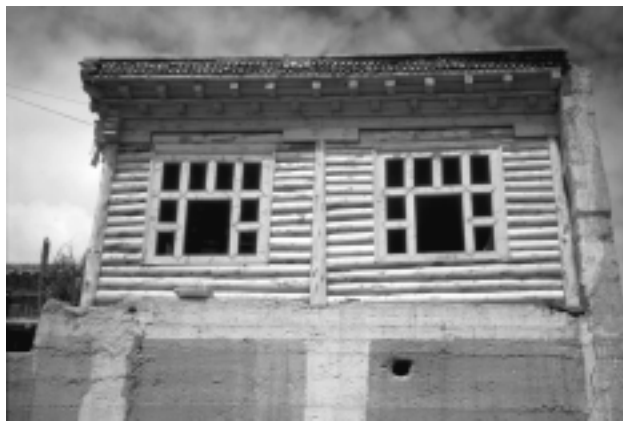
FIGURE 12. Ad-hoc use of “modern products”: glass bottles fill the eave area traditionally occupied by timber, brush or slate. (Photo by author, 1999.)
