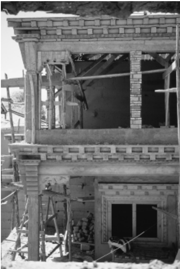
FIGURE 9. Hybrid construction on a new house in Dengke. Rammed-earth walls enclosing new poured concrete, brick, and timber wall structures. (Photo by author, 1999.)
