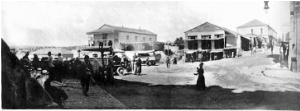
Jaffa Gate, the present condition, showing the market sprawling over the road area and upon the Fosse (now covered).
