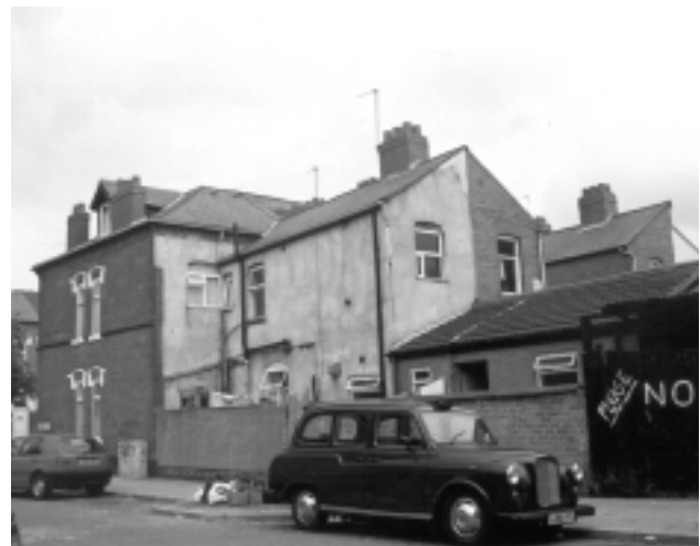
FIGURE 5. The terrace house has typically experienced expansion to the rear of the plot and in two-story extensions, as well as attic and cellar conversions.
