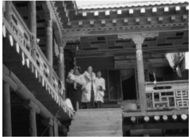
FIGURE 10. Recently completed lov benka house that conforms to the image of a local tradition accepting of new materials and products. Thus, the concrete steps take the place of timber or earth steps, and Chinese clay tiles appear at the edge of the roof. In addition, the square timber ends running under the eaves are probably of imported, bought softwood, unlike the round-ended locally available timber that supports the floor of the upper level. (Photo by author, 1999.)
