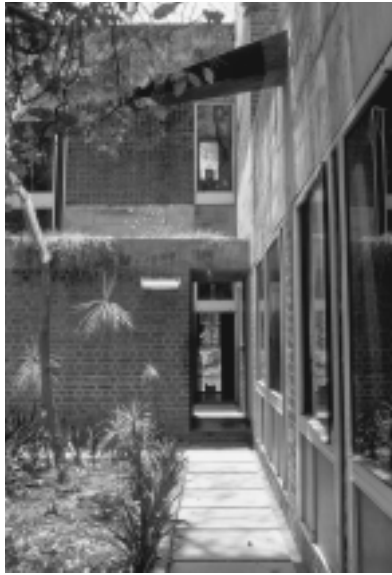
FIGURE 10. Northeast dining room and living room win- dows receive early morning sun in May.
