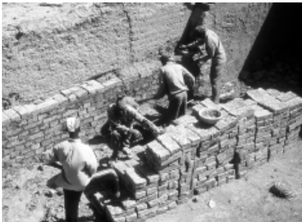
FIGURE 9. A coordinated arrangement of laborers who pass materials onto an apprentice setting brick courses for a new wall.
