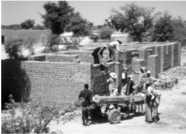
FIGURE 3. Construction site of a new house along the Bani River.
