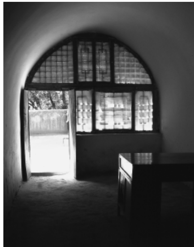
FIGURE 6. This image shows the muted quality of light that typical of a traditional yaodong, lit only through the arched front opening.
