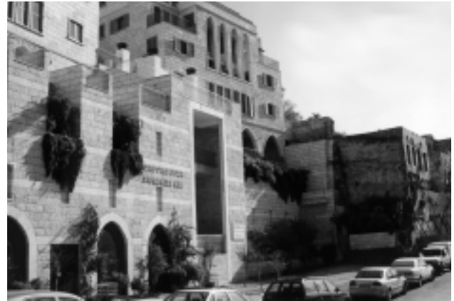
FIGURE 8. West facade of Andromeda Hill.
