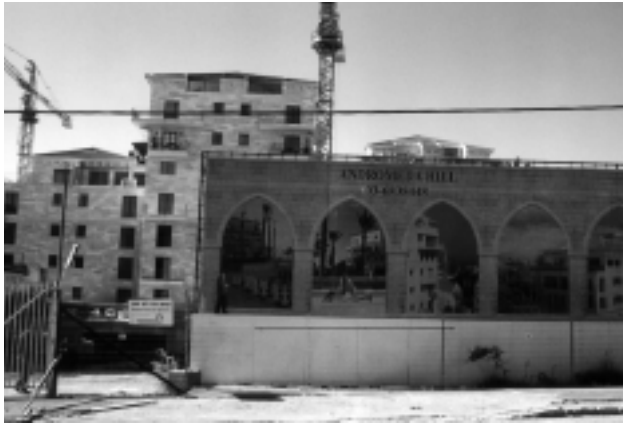
FIGURE 7. East facade of Andromeda Hill, seen from Yefet Street.
