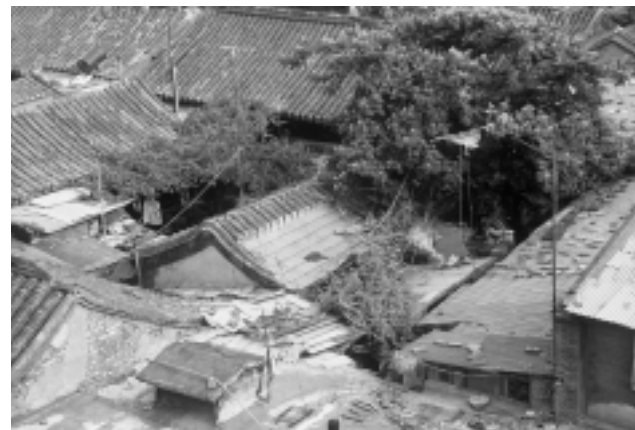
FIGURE 3. A courtyard house in a typically dilapidated and crowded condition. Most of the open courtyard space is filled with “temporary” shelters, kitchens, and storage sheds.
