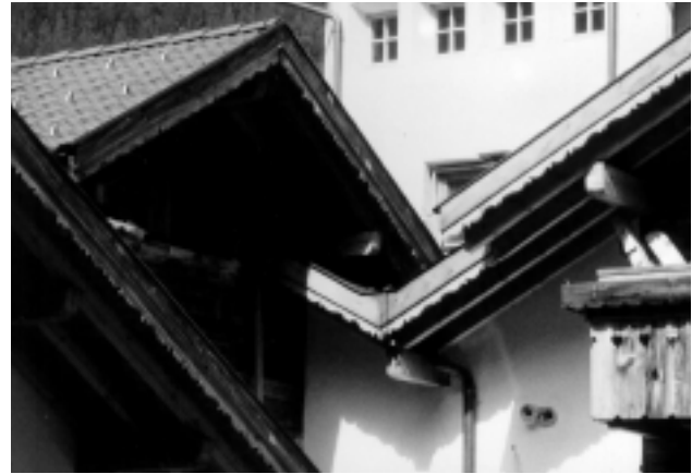
FIGURE 8. (RIGHT) The higgledy-piggledy arrangement of chalet gables bears little structural relation to the underlying concrete cube.
