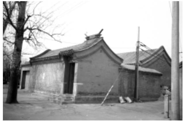
FIGURE 12. A privately rebuilt siheyuan on its original plot within the Shishahai preservation district. Note the garage door on the left.
