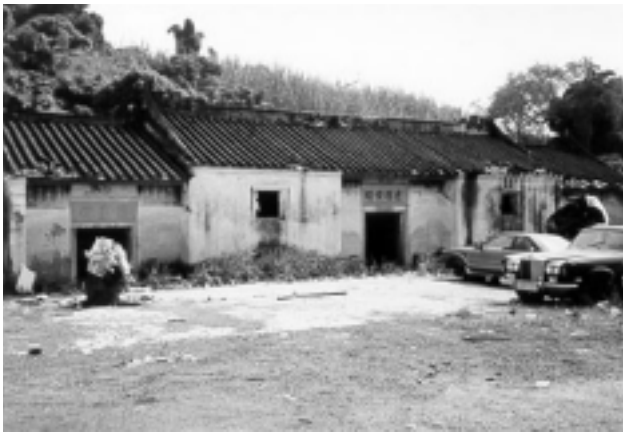
FIGURE 1. (TOP) The flooded hall. (Photo by author.)
