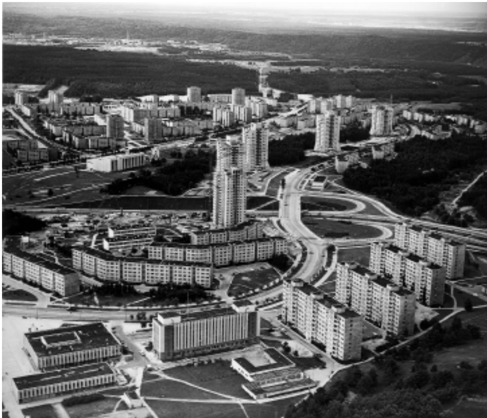
FIGURE 8. Aerial view of Lazdynai outside Vilnius, designed by Vytautas Čekanauskas and Vytautas Brėdikis (constructed 1964-1972; twenty-story towers added in 1982). (Source: author’s collection.)
