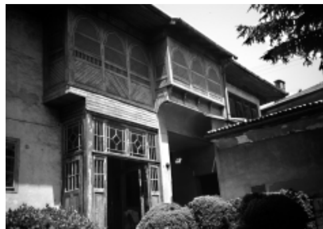
FIGURE 8. Elevated open-air porch (doksat), with mushebak screens.
