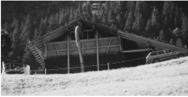
FIGURE 5. A new barn is built using frame construction, with the outer wall being “overclad” with logs. Gsteig.
