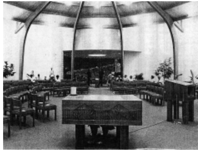
FIGURE 14. Saint Benedict the African Church, Chicago, IL. The ceiling system reflects the traditional hut form and uses wood decking to emphasize its circular form. (Source: St. Benedict Building Planning Committee.)
