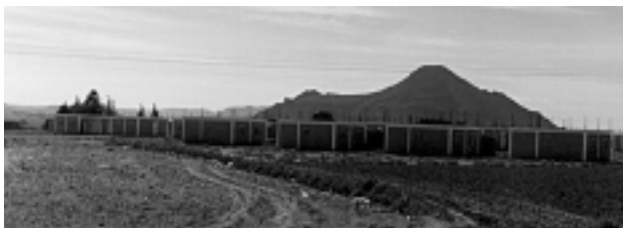
FIGURE 20. "Earthquake housing," Al Wasta, Ma'bar, 1990.
