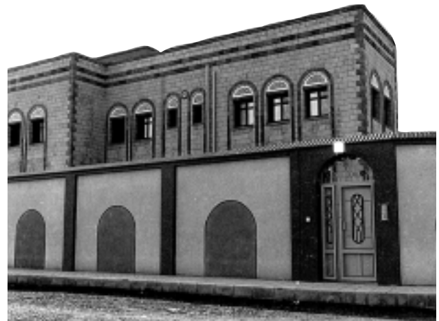
FIGURE 11. Villa in Sana'a, completed in 1990, with stone for the building and concrete blocks for the yard walls.
