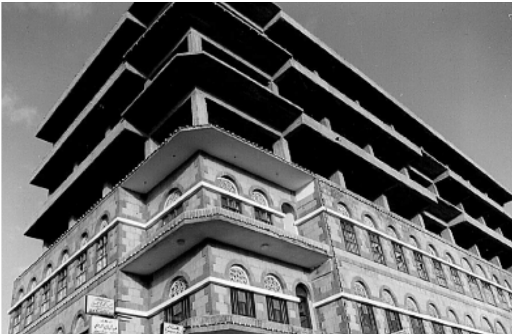
FIGURE 12. Concrete frame and stone facing in construction, Sana'a, 1990.
