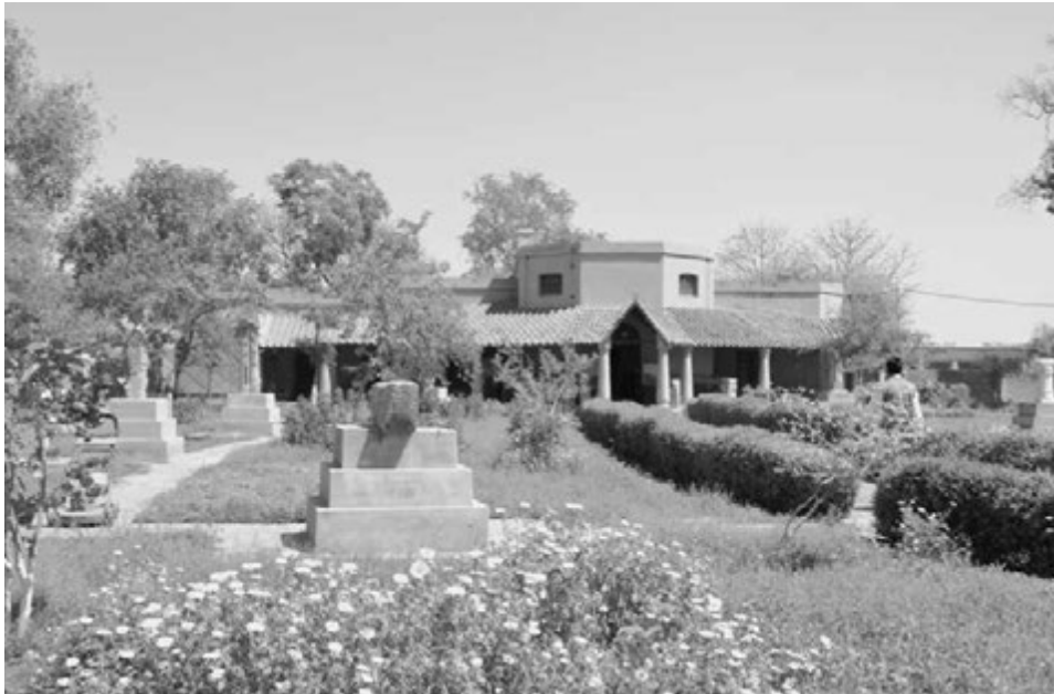
FIGURE 12. Thomas's Jahaj Kothi. View of the front garden and main house. Photo by author.
