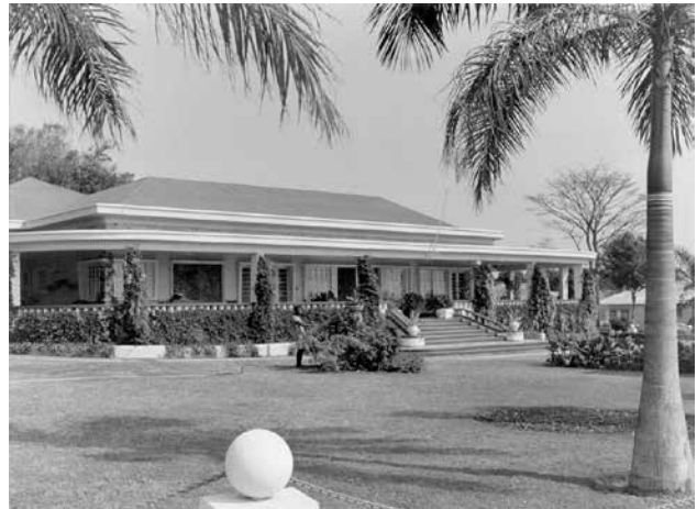
FIGURE 12. Diamang’s Representation House, K-18, is used today by the board of directors of Endiama, the Angola National Mining Company. Courtesy of diamang.com .
