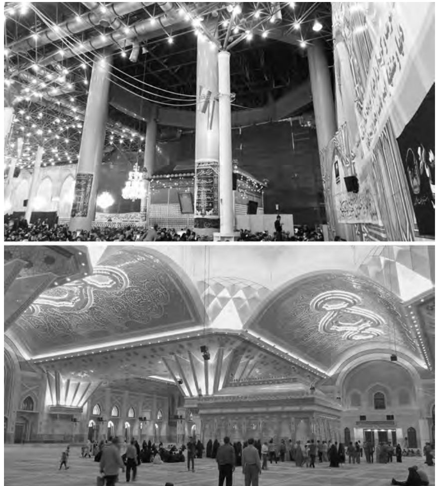
FIGURE 12. Interior design of the mausoleum-shrine of Ayatollah Khomeini. Above: after the initial phase of construction (1991) eight columns surrounding the burial space carried the weight of the main dome. Below: after the second reconstruction phase the interior was vastly expanded and the dome was raised to create a new ceremonial space. Top image from the author’s personal collection. Bottom source: Wikimedia, retrieved from https://upload.wikimedia.org/wikipedia/commons/ff/f4/Mausoleum_of_Ruhollah_Khomeini_07.jpg .
