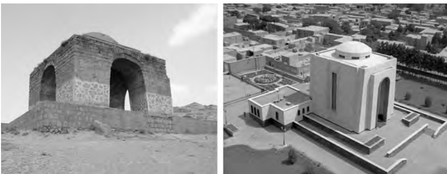
FIGURE 9. The Persian concept of châhâr-tâq. Left: a Zoroastrian fire temple (atashkadeh) at Niasar, Kashan, in which four heavy piers with joined arches carry the weight of a dome to create a simple pavilion. Right: employment of the châhâr-tâq idea in the design of the mausoleum of Reza Shah. Left image from the author's personal archive. Right image from the 1978 Albert Lamorisse documentary video The Lovers' Wind .
