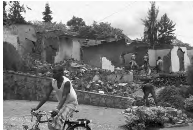
FIGURE 15. Demolition of an informal neighborhood in Kigali, Rwanda. Photo by author, 2017.
