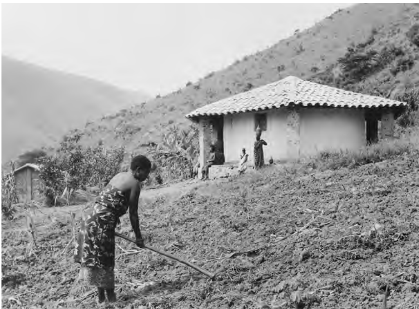
FIGURE 7. This round dwelling matches the description of the first kind of house to be built in 1947 as part of a colonial housing program: circular in plan, but constructed with solid materials (bricks, stones, and tiles). Source: Collection RMCA Tervuren; photo J. Mulders (Inforcongo), RMCA Tervuren ©.
