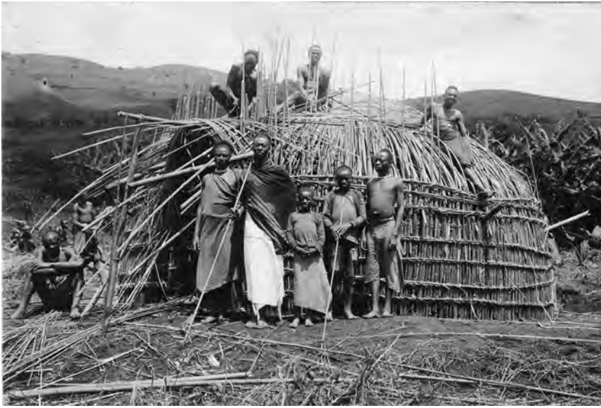
FIGURE 4. Construction of a Tutsi dwelling in Rwanda. Source: Collection RMCA Tervuren; photo Provost.
