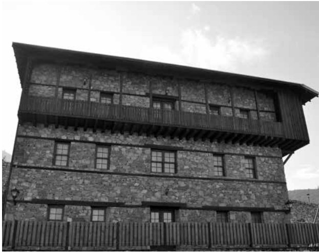
FIGURE 20. The Struga house built in the Macedonian Village. Source: author's archive.
