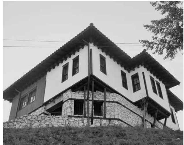
FIGURE 15. The "Veleshka" house in the Macedonian Village. Source: author's archive.
