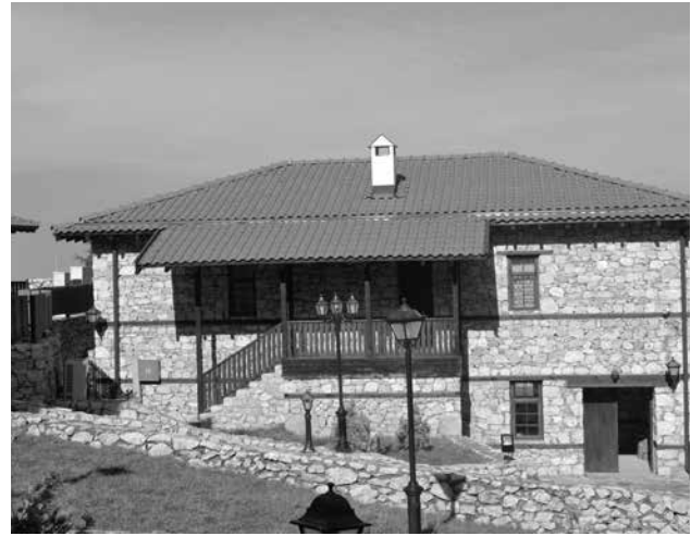
FIGURE 17. The entrance view of the house representing the Bitola region. Source: author's archive, 2014.
