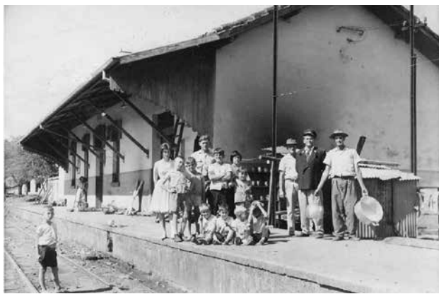
FIGURE 13. The Cosmópolis station in the 1960s. Source: Archive of the Centro de Memória de Cosmópolis.
