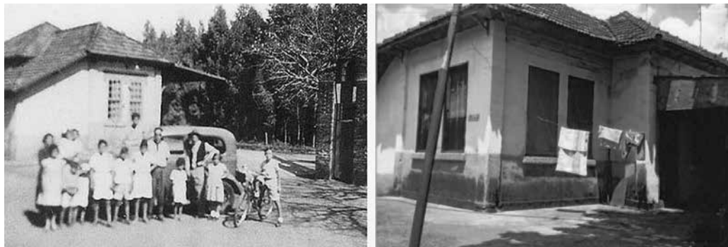
FIGURE 9. Santa Genebra Station, Barão Geraldo, 1950 (left) and 2011 (right). Source: www.estacoesferroviarias.com.br .
