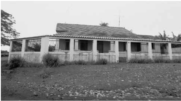
FIGURE 16. The old building of the Guaiquica Farm in 2014. Source: group's research archive.
