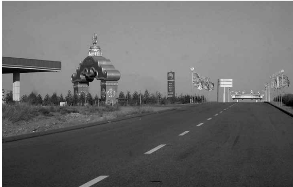
FIGURE 9. Ordos infrastructure, clad in theme-park aesthetics, stretches anticipation for the sedentarized monument across the landscape. Photo by author, 2009.
