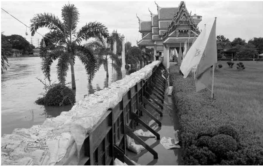
FIGURE 10. Temporary and localized approach to flood risk protection continues to be the norm today. Source: Fine Arts Department.
