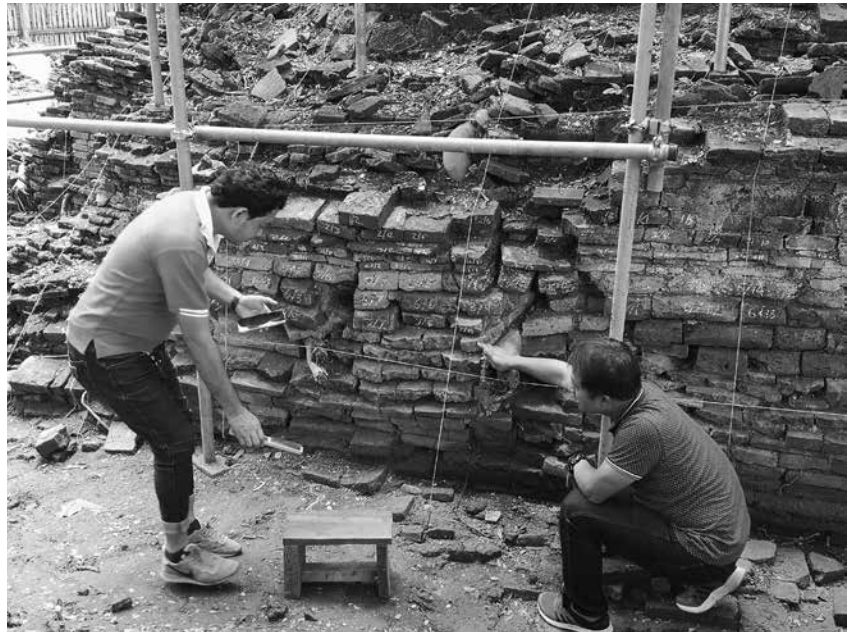
FIGURE 11. During pilot training at an ancient monument in Ayutthaya, specialists engaged in detailed documentation of individual bricks in the plinth, suggesting this historical profile would be retained (June 2019). Source: https://www.facebook.com/RakWatKrachee/
