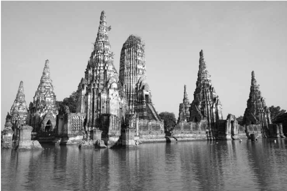
FIGURE 5. Prolonged flooding at the iconic Wat Chai Wattanaram in 2011. Photo by author.
