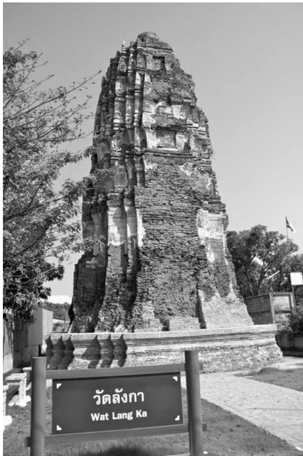
FIGURE 8. Example of a post-flood restoration project, with new plastering and landscaping. Photo by author.
