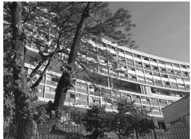
FIGURE 18. Block A with new aluminum windows painted in blue, 2016. Photo by author.
