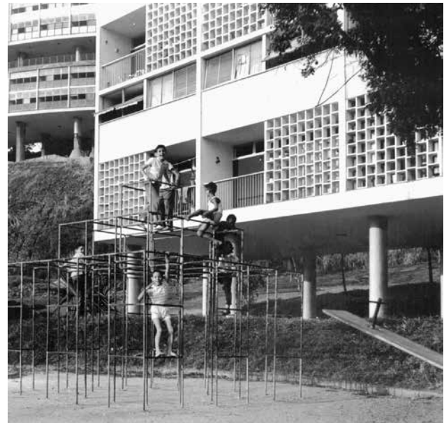
FIGURE 13. Playground area next to Block B apartment building, c. 1950. The cobogó panels can be seen. Source: Arquivo Geral da Cidade do Rio de Janeiro.
