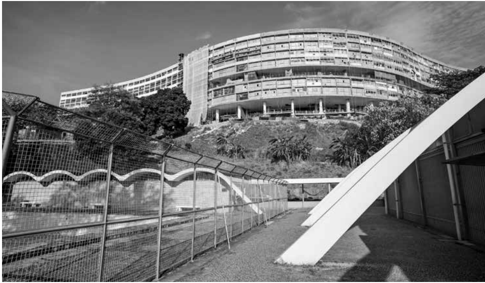
FIGURE 16. Block A under renovation, 2014. Photo by Alfredo Britto.
