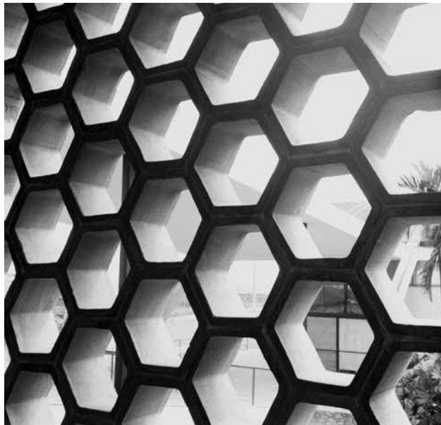
FIGURE 2. Cobogó panel in the school building, c. 1950. Source: Centro de Documentação Syvio de Vasconcellos, UFMG.
