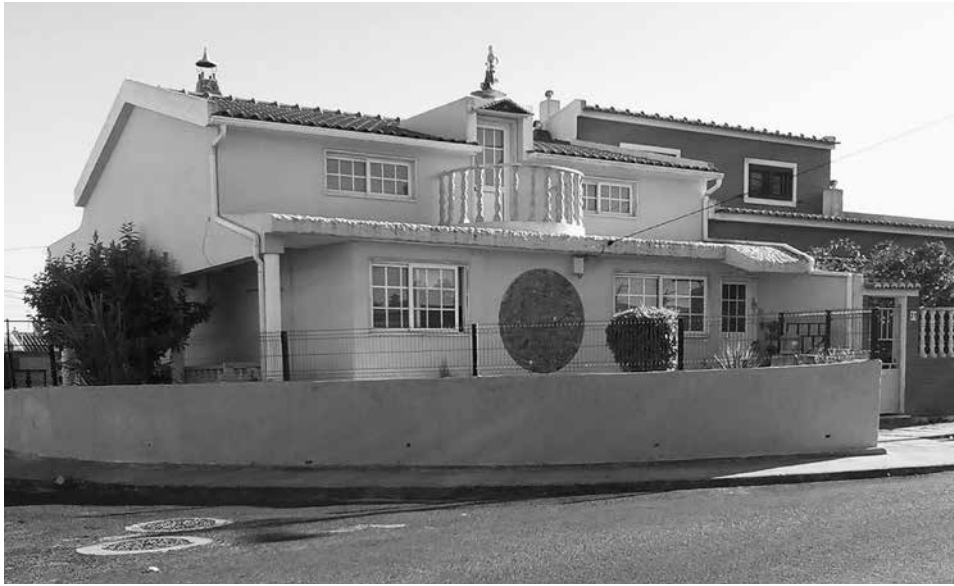
FIGURE 10. Prefabricated CAR house, cement model, as it appears today in Camarate, Lisbon. Based on: Joana Gouveia Alves, July 2017.
